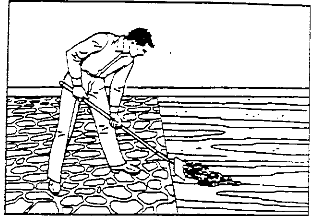
Sketch 13. Stand on the remaining floor covering, not the felt, during felt removal.
