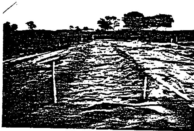
Fig. 19 View showing trenches in sand. These can be placed using a crawler tractor with blade. A wheel tractor will not work.
