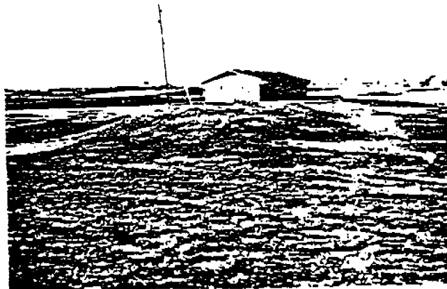
Fig. 24 View of finished mound prior to final hand leveling and seeding.
