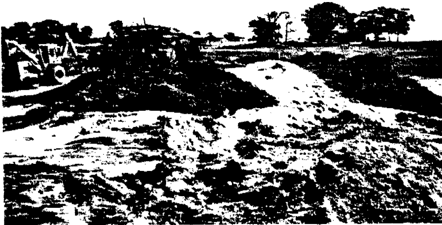
Fig. 23 Placement of topsoil on mound. Note layer of hay or straw on top of rocks prior to placement of soil. Blade on crawler is superior to bucket for leveling. Tractor with wheels should not be used, as it ruts up the mound too much.
