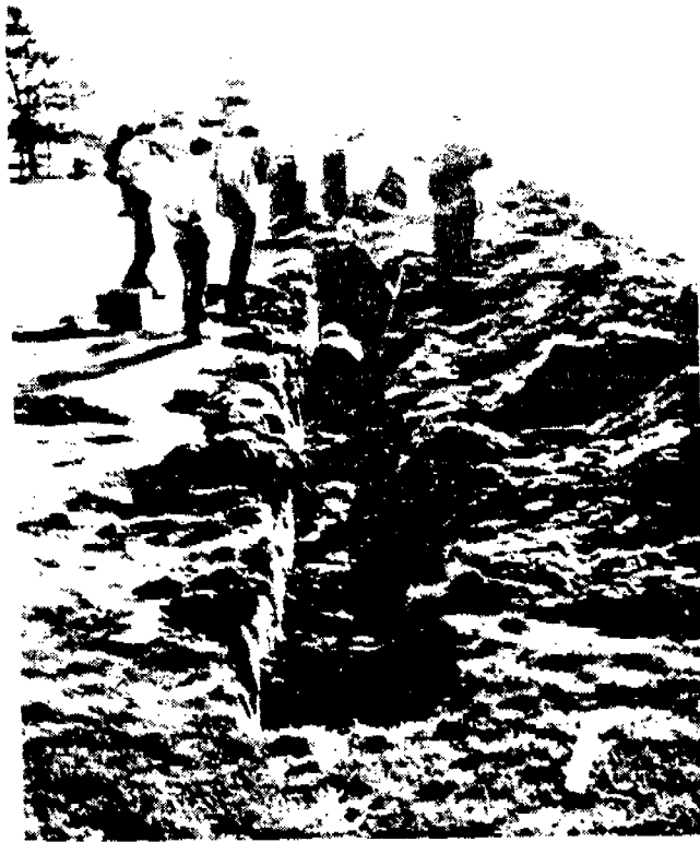
Fig. 15 Trench and lay the pipe from the pumping chamber to the mound system. Refill trench and compact soil to avoid settling under mound.
