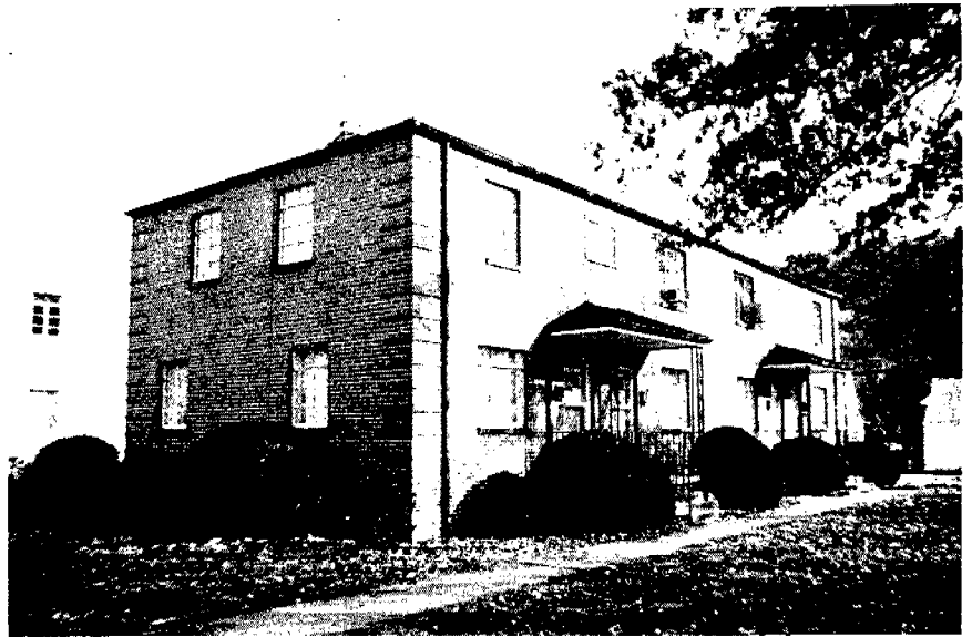
Garden Apartment (211) C Use Code 011 Construction Type 1
