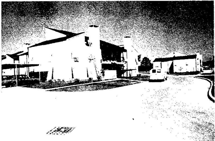
Garden Apartment (211) C- Use Code 011 Construction Type 1
