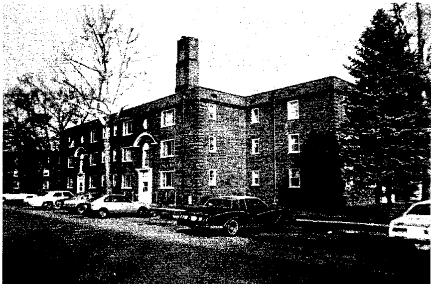
Garden Apartment (211) C+ Use Code 011 Construction Type 1
