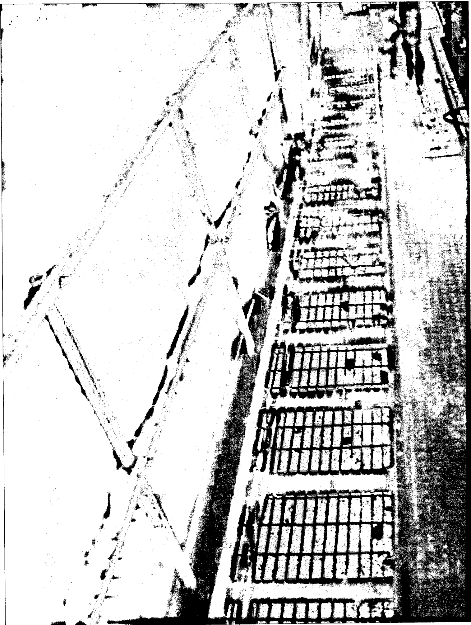
403 CAR RUN WALKWAY ADJACENT TO CONVEYOR
